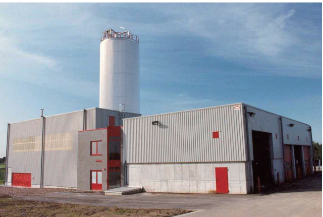
Brecht Organic Waste Dry Anaerobic Project, Belgium. Capacity 140 tons/day. (2000)
