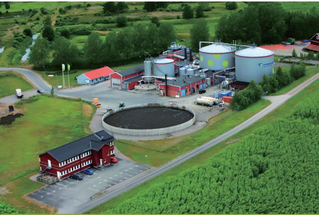
Linköping Organic Waste Biogas Plant, Sweden. Capacity 270 tons/day. (1996)
