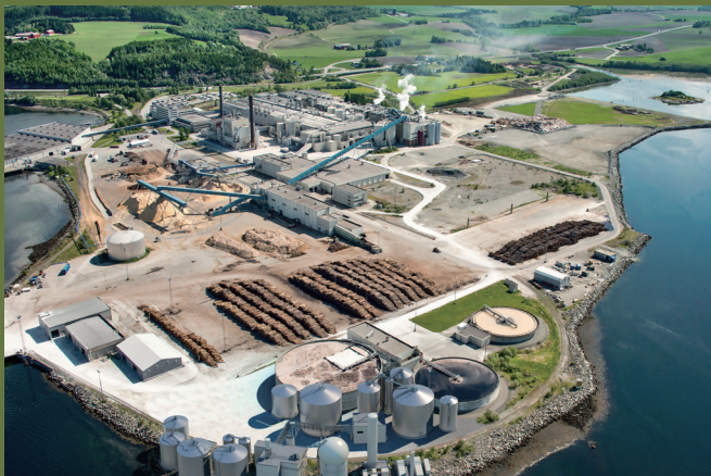
Biokraft Biogas Plant, Norway. (2017)
