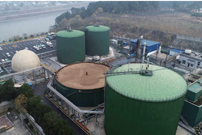
Changsha Food Waste Treatment Project. Capacity 800 tons/day. (2014)
