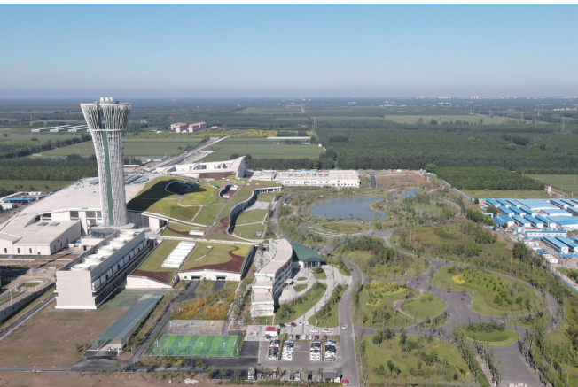
Xiong'an Integrated Waste Treatment Facility Phase I Anaerobic Project, Hebei. Capacity 600 tons/day. (2024)
