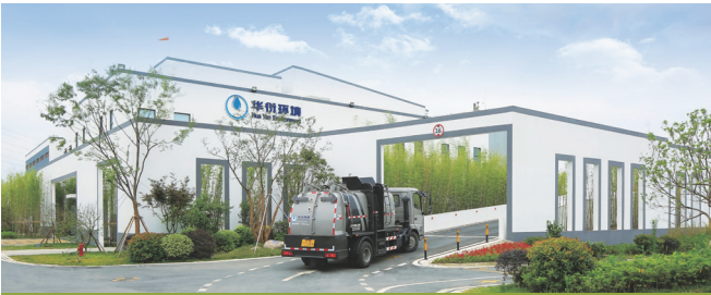
Suzhou Industrial Park Food & Green Waste Treatment Phase I Project. Capacity 400 tons/day. (2018)
