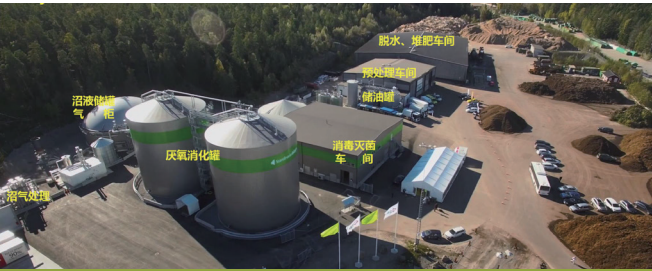
Södertörn Biogas Plant, Sweden. Capacity 110 tons/day. (2014)
