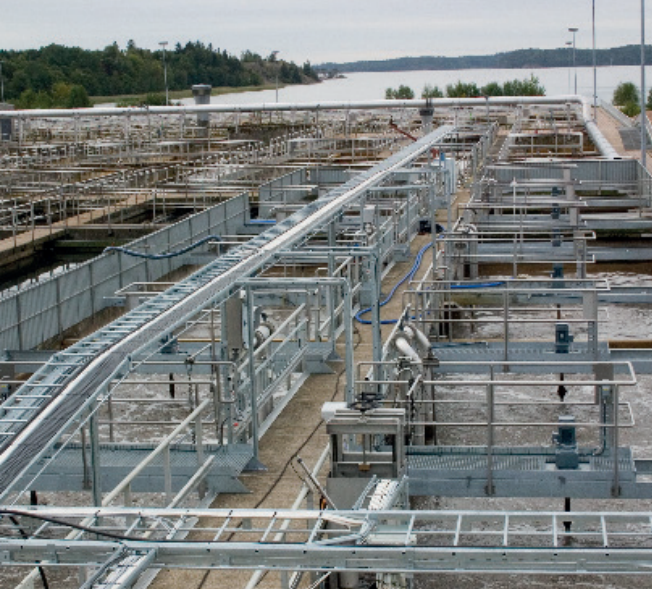
Himmerfjärden WWTP, Sweden. Capacity 480 kgN/d. (2007)
