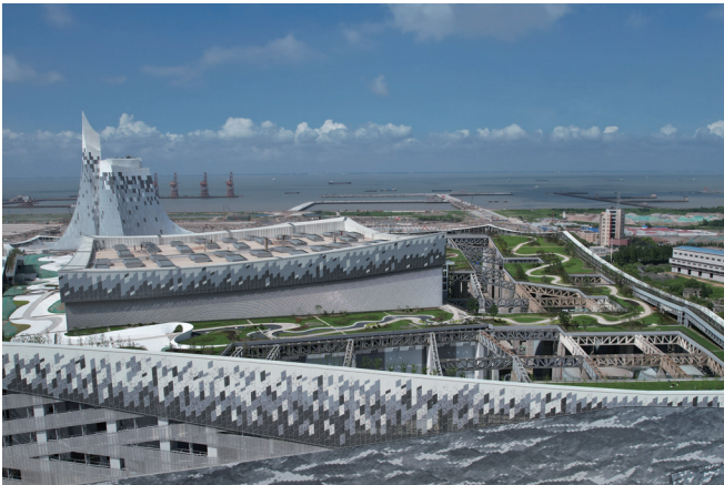
Baoshan Renewable Energy Utilization Center Wet Waste Treatment Project, Shanghai. Capacity 800 tons/day. (2023)
