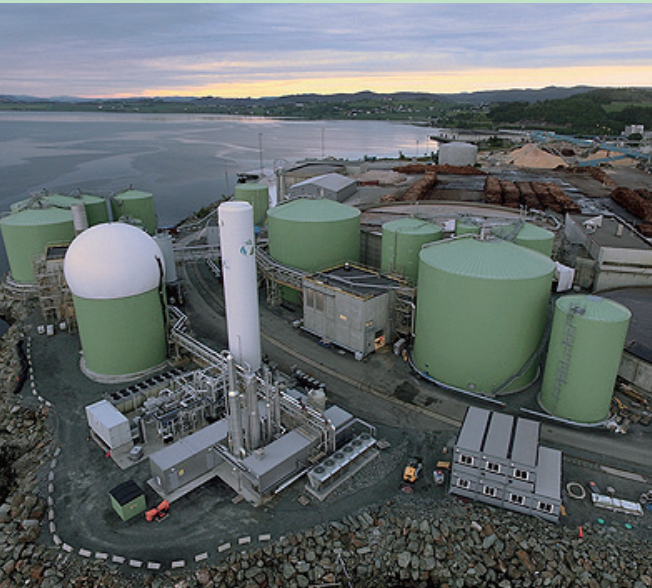
Biokraft Aquaculture Waste Treatment Project, Norway. (2017)
