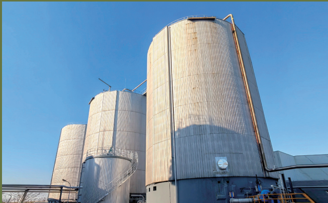
Dongcun Sorted Waste Comprehensive Treatment Food & Kitchen Waste Anaerobic Retrofitting Project, Beijing. Capacity 550 tons/day. (2023)
