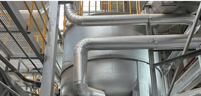
Dongcun Classified Waste Comprehensive Treatment Food Waste Pretreatment and Anaerobic Reconstruction Project, Beijing. Capacity 550 tons/day. (2023)
