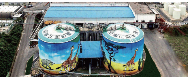
Heishizi Food Waste Phase I-IV Treatment Project, Chongqing. Capacity 1000 tons/day. (2012)
