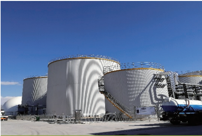
Tongzhou Urban Organic Waste Co-Anaerobic Treatment Project, Beijing. Capacity 600 tons/day. (2018)
