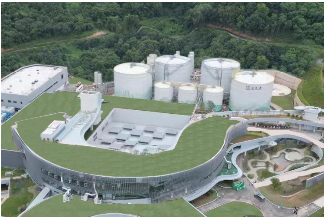
Guangming Environmental Park Food & Kitchen Waste Treatment Project, Shenzhen. Capacity 1000 tons/day. (2023)
