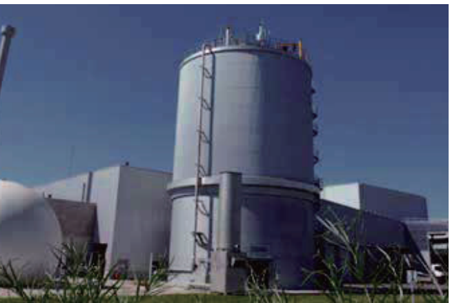
Bourg-en-Bresse Mixed Waste Dry Anaerobic Project, France. Capacity 110 tons/day. (2015)
